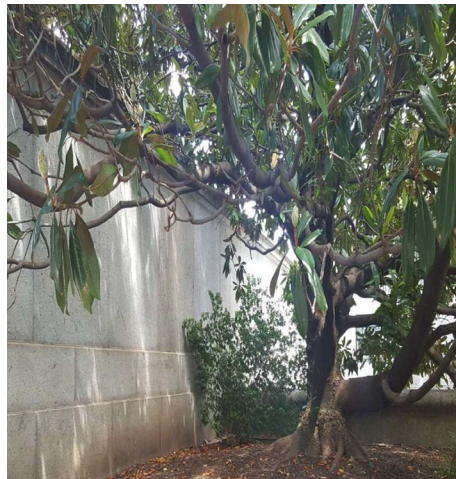
Photo 1 East Side of 11'6" Wall
