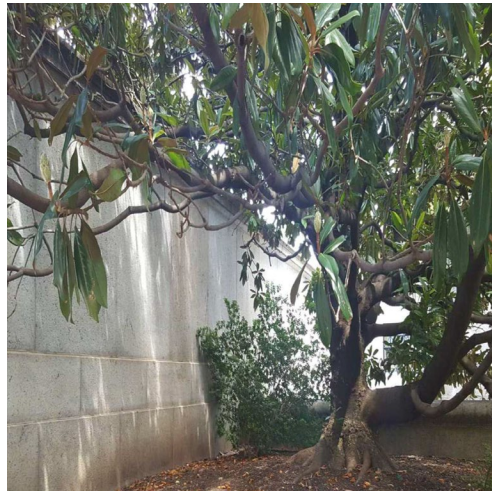
Photo 1 East Side of 11'6" Wall
